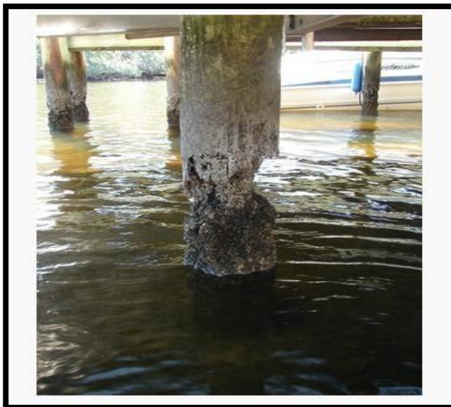
Fig 1.18: Alkali aggregate reaction on concrete
