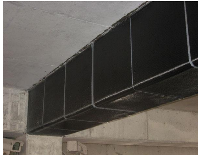
Fig 3.9: Placing of carbon fibre to the beams
