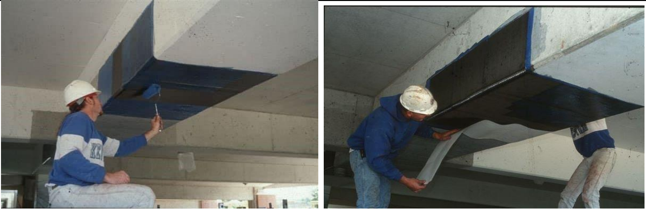
Fig 4.3: Strengthening with FRP laminates
