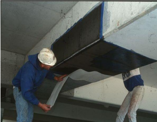
Fig 3.9: Placing of carbon fibre to the beams
