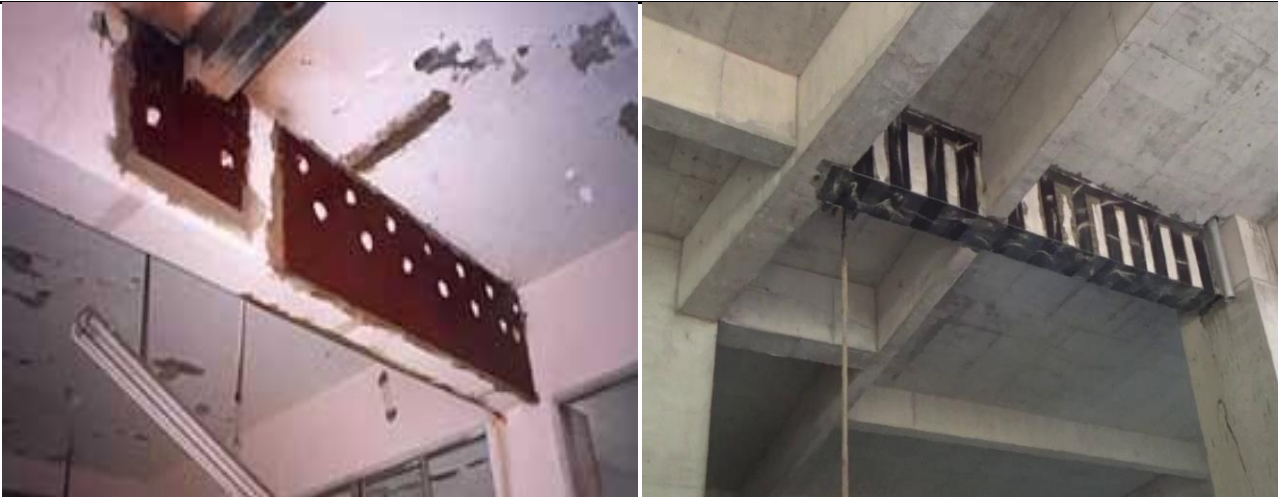
Fig 4.2: External bonding by mild steel plates
